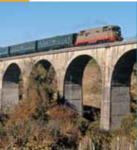
Faentina railway near the Borgo San Lorenzo Station
